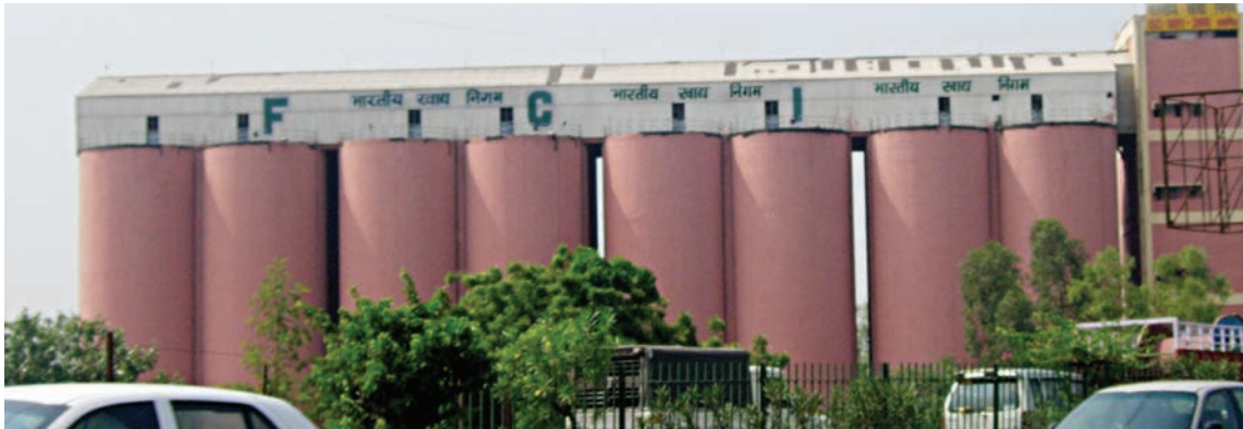
Fig. 1.10 (a) : Silos for storage of grains
